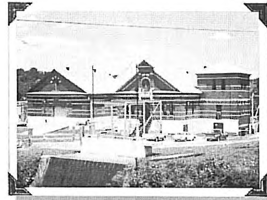
The historic Waterworks plant has been in operation since 1899, providing drinking water for area residents. Canal water is also a source of hydropower, with the City committing water revenue to the ACA.
